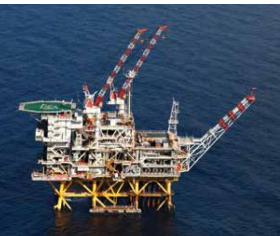
Vega Oil Field – “Vega A” production platform and “Leonis” FSO Offshore Sicily
